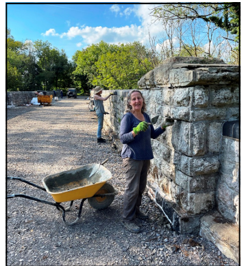
Laying the coping. Note the improvised hoist.
