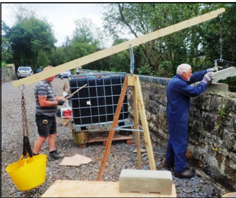
Laying the coping. Note the improvised hoist.
