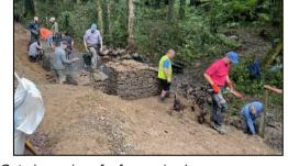
Gated crossings for farm animals were constructed in concrete at four locations (to prevent damage to the path) and considerable clearance and fence building was carried out in the wooded section. The stone in a railway masonry retaining wall alongside the path was spalling and in need of pointing (illustrated); this provided a feature for users to enjoy.
